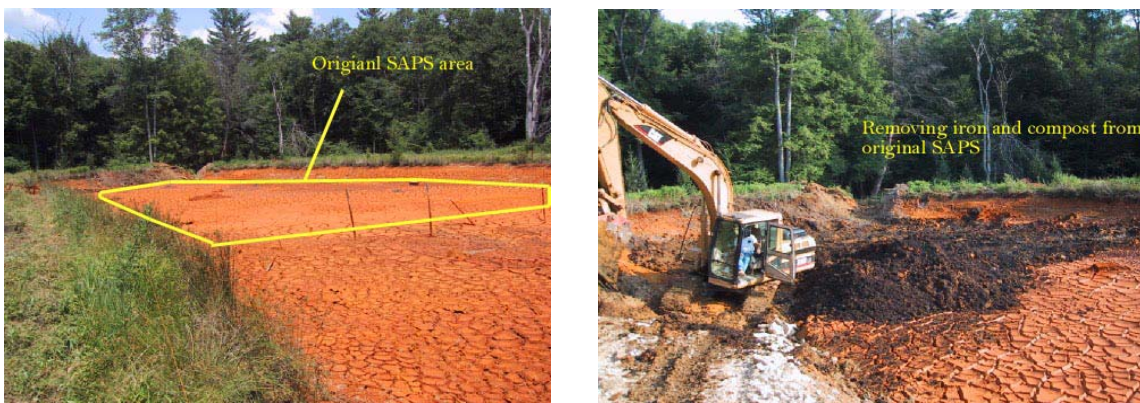
Figure H3 & H4. SAPS reconstruction at Howe Bridge in 2002, Corsica, Pennsylvania.
