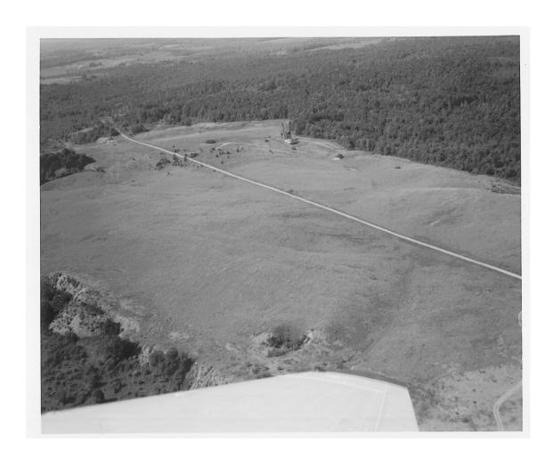
Figure 1. Aerial View of Mine Site 33 in the Gilmore Run Subwatershed of Big Scrubgrass Creek Watershed. Most of this mine has been adequately reclaimed to prevent acid mine drainage pollution. The recommendations in this report are aimed at achieving acid source abatement for all sources within the watershed.
