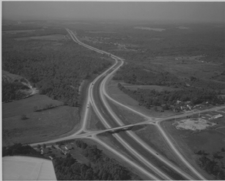
Figure 4. Aerial view looking west along Interstate 80 at the Clintonville Interchange in the Big Scrubgrass Creek Watershed. This highway intersects with Interstate 79 west of the watershed providing excellent access to the area from major population centers, which should help promote future economic growth in the area.
