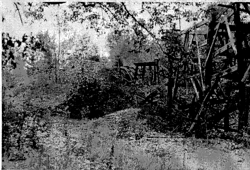
Figure 11. Remains of a deep mine operation in the Southwest Tributaries area south of the Village of Nectarine. The portal has been obliterated by later strip mining on the hillside. Runoff from gob piles on the surface is a source of stream pollution.
