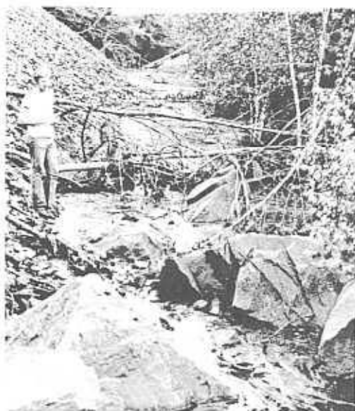
GREENWOOD-EAST REFUSE SEEPAGE
