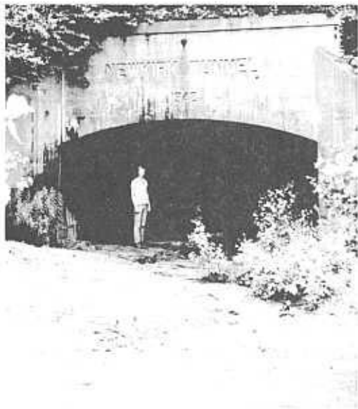
NEWKIRK MINE PORTAL
