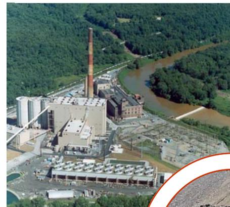
*The CFB power plant in Seward, Penn. is the largest waste-coal plant in the world, and was built atop coal refuse and CFB ash.*
